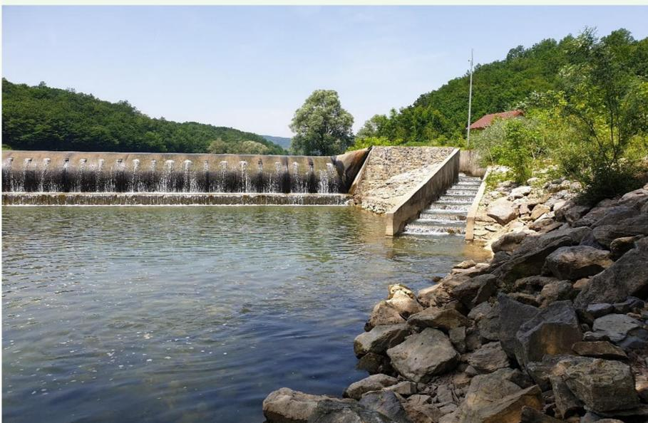
Figure 2. Fish passage in function on MHE Ilovac.
